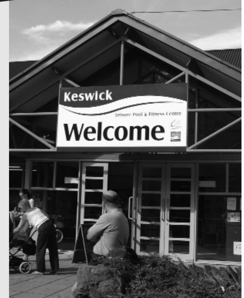
Entrance to Keswick Leisure Pool
